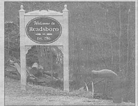
Readsboro's new dry hydrant.
