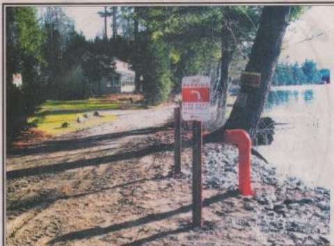
PREPARING FOR FIRE—The Newbury Fire Department installed this dry hydrant on Hall's Lake on Nov. 18.
